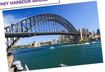
SYDNEY HARBOUR BRIDGE
